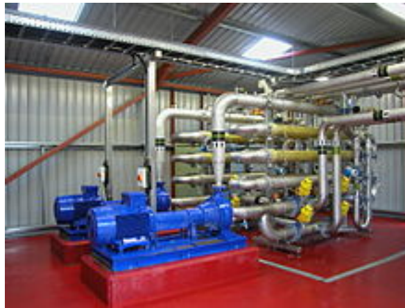
UF membrane side stream configuration
