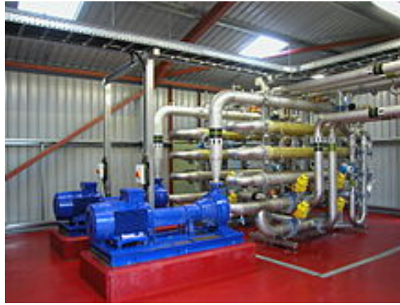
UF membrane side stream configuration
